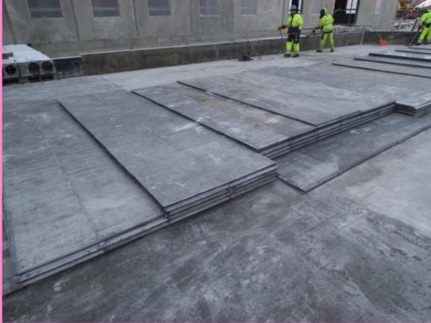
05.02.14 at Tartu University Hospital bunker construction
